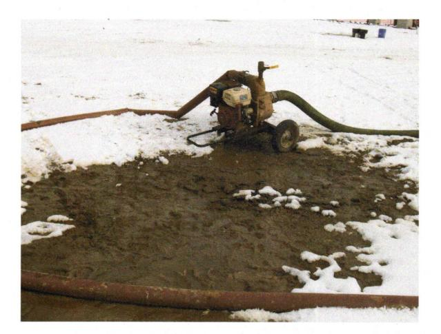
Description: Frac Flow Back Spill at Storage Tanks – note the lack of pollutional substance containment measures.
