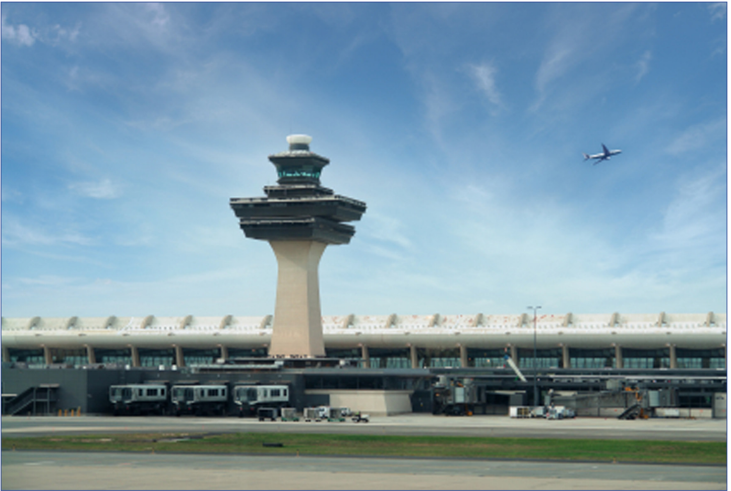
Washington Dulles International Airport main terminal and control tower.
