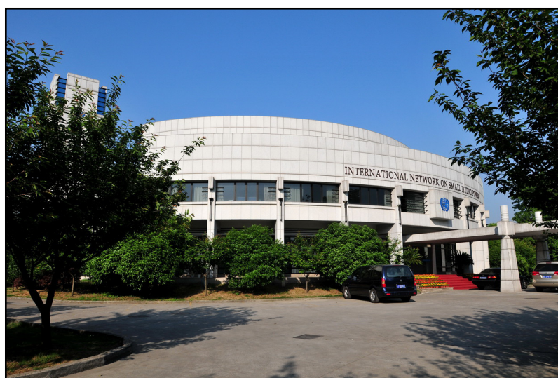
Fig. 11: The IC-SHP building in Hangzhou, China
