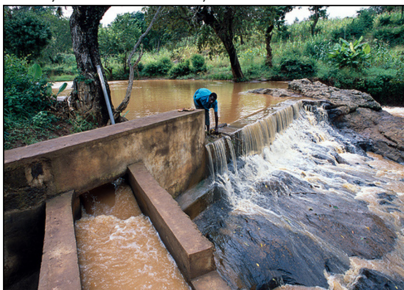
Fig. 14: Weir of the Tungu-Kabri project, Mbuiru, Kenya. The project was funded by the UNDP and developed by Practical Action East Africa and the Kenyan Ministry of Energy. Source: Practical Action
