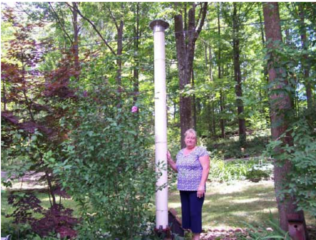
After Julie and Craig Sautner leased their land to Houston-based Cabot Oil and Gas Corp., the company's improper drilling contaminated their water. Julie Sautner stands next to a vent that allows natural gas to escape from their water well so their home will not explode.
