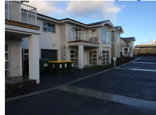
Greenwich Gardens – Stage 1 Villas shortly after completion.
