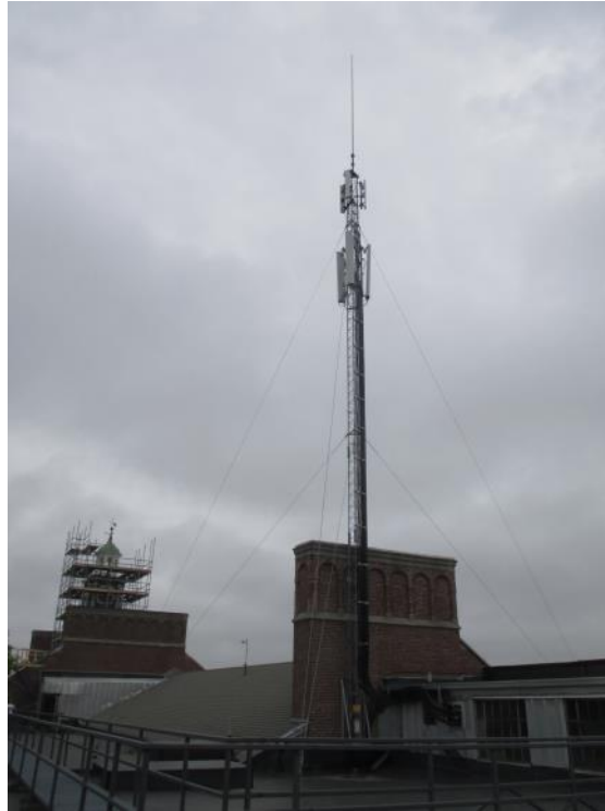
Figure 1: City of Portland / U.S. Cellular Guyed Tower
