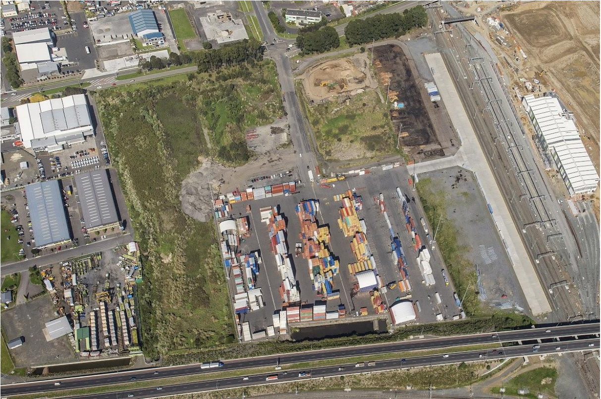
Figure E: Wiri Inland Terminal (viewed from the north)
