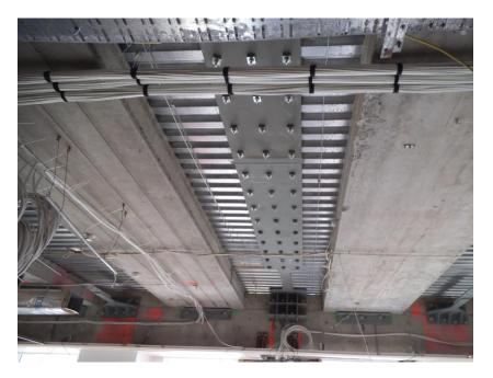
Tower floors strengthened with 457 tonnes of structural steel fastened by 5,000 bolts, 25,000 anchors and 11,800 metres of post-tensioning strand
