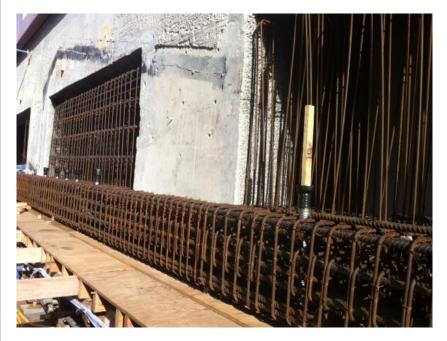
Transfer beam strength improved with the addition of 74 tonnes of reinforcing steel and 194 cubic metres of concrete
