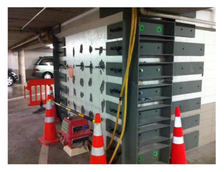
Shear core strengthened with the addition of 727 tonnes of structural steel, fastened by 15,000 bolts and 8,500 anchors
