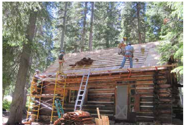
Replacing the roof on the historic Cascade Canyon Patrol Cabin.
