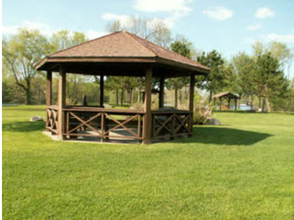
The gazebo should be relocated to another site within the Town.
