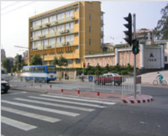
Figure B10.6.2 Staggered Pedestrian Crossing
