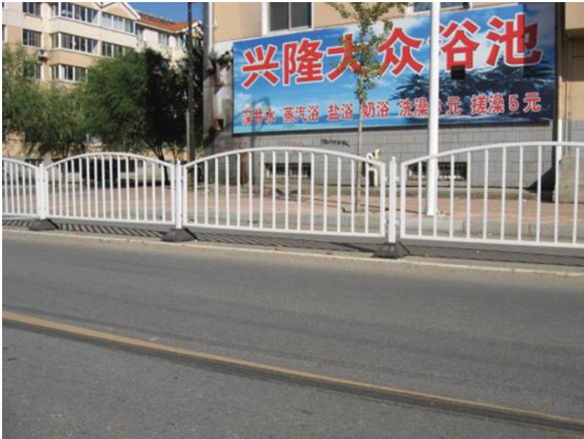
Figure 10.6 Lane Separators in Jinzhou, Liaoning
