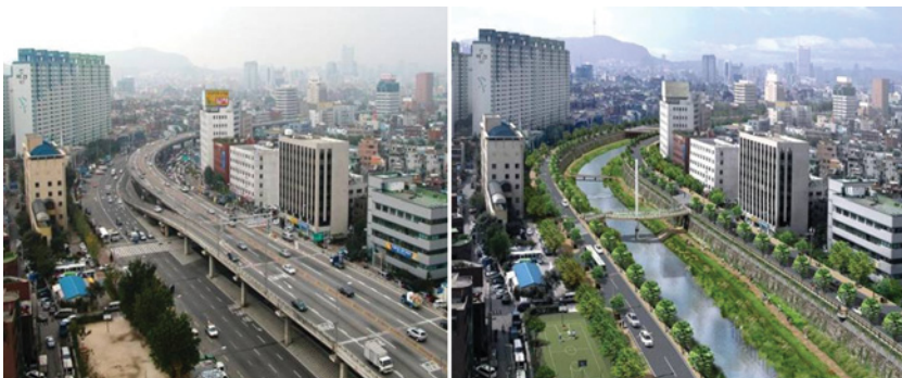
Figure 12.3 The Cheonggye and Samil Elevated Highway (Left) in Seoul Was Demolished in 2003 and Replaced by a Restored Cheonggye Stream (Right)
