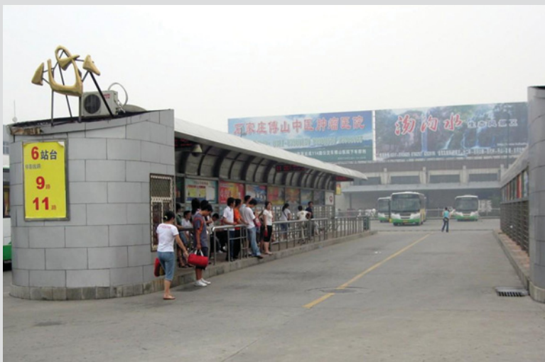
Figure B11.5.1 Bus Interchange Terminal in Shijiazhuang
